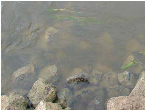
Figure 19: Techno-lithal (rip rap)
