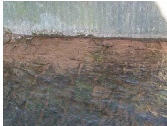
Figure 20: Techno-lithal (stone plastering)
