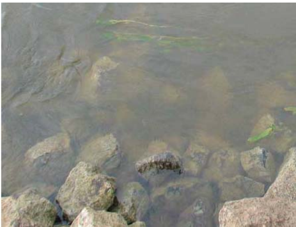
Figure 19: Techno-lithal (rip rap)
