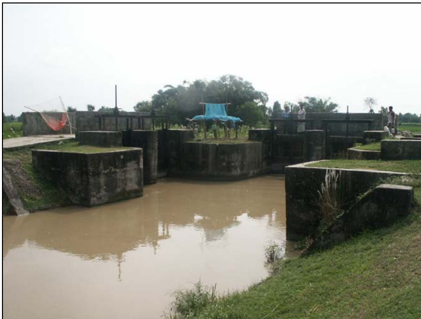
Figure 9: N01BG011: Nepal - Bagmati Canal - Malahi, upstream of barrage
